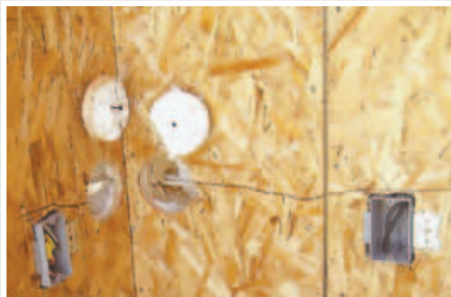
EPS SIPs package includes pre-assembled, factory-insulated headers, along with window and door cutouts and horizontal and vertical electrical chases (if requested.)
