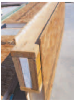
EPS SIPs package includes pre-assembled, factory-insulated headers, along with window and door cutouts and horizontal and vertical electrical chases (if requested.)
