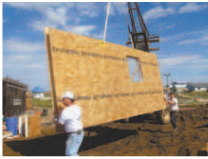
Jumbo 8' x 24' panels can make construction much faster.
