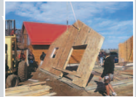
Field pre-assembled wall options are solid and fast.
